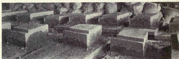
FIG. 38—DIMENSION STONE ON PLANK PALLETTS SUPPORTED ON BANKERS. NOTE WIDE "RETURN" OF WHITE FACING
